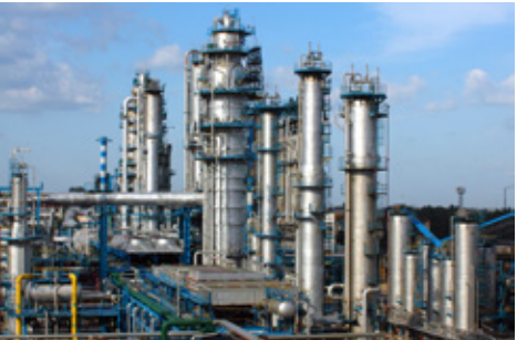
Petroleum, chemical industry
